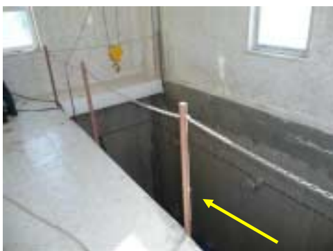
Picture 5.1 Situation at Kepez
