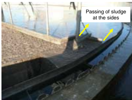
Picture 3.14 Skimmer for removal of the floating layer
