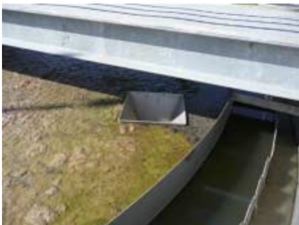
Picture 4.9 Floating layer removal device
