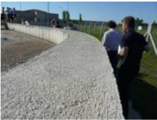
Picture 3.11 Thick walls of activated sludge tanks
