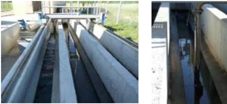
Picture 3.2 Sand removal construction (1)
