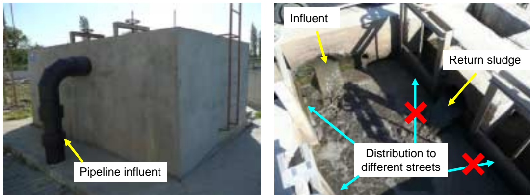
Picture 3.6 Distribution construction
