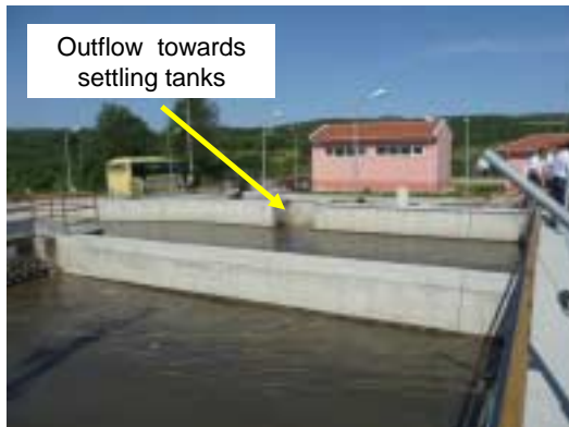
Picture 4.6 Activated sludge tank
