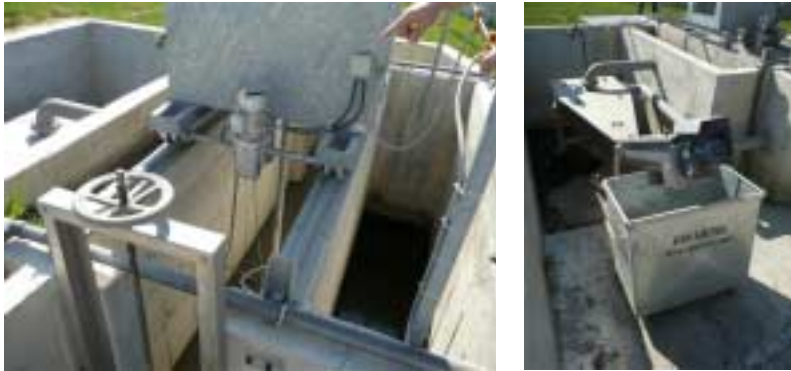
Picture 4.3 Sand removal construction
