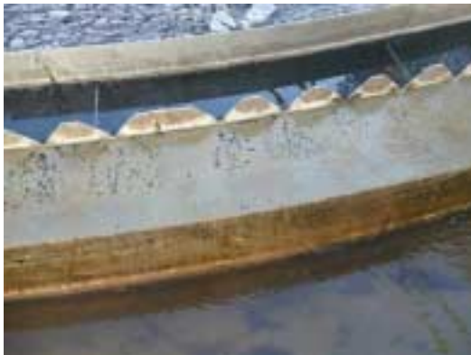
Picture 3.15 Edge of overflow of settling tanks + return sludge basin
