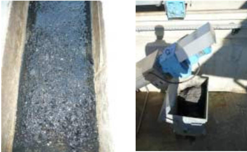
Picture 3.3 Sand removal construction (2)
