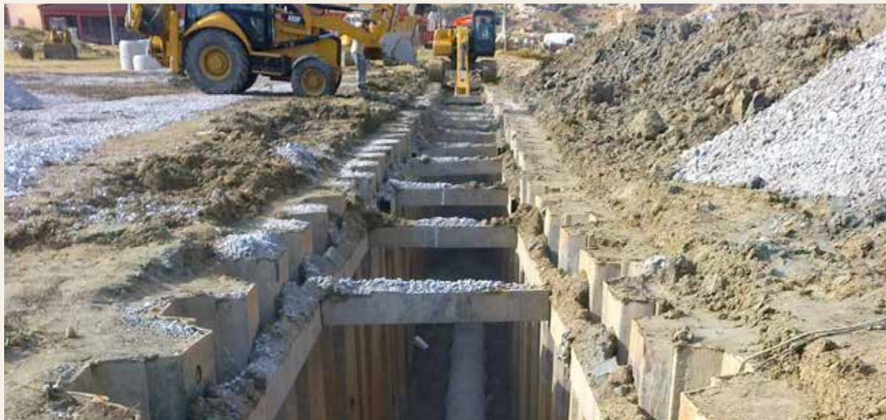
Aydin / Sazli, Sewer Construction
