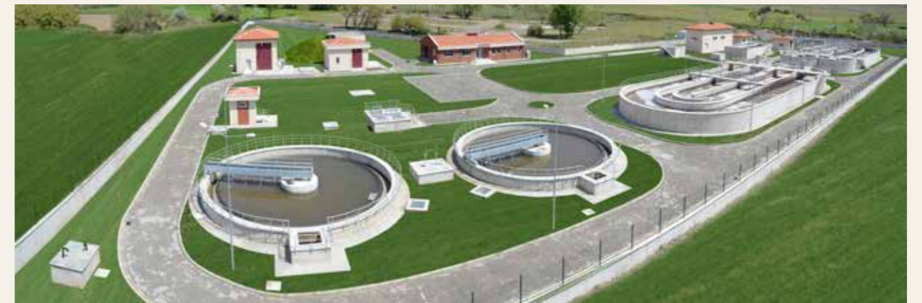
Corum / Iskilip, Wastewater Treatment Plant
