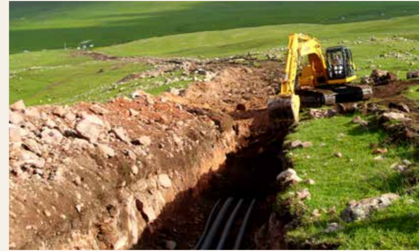
Ardahan/Köprülü, Potable Water Construction
