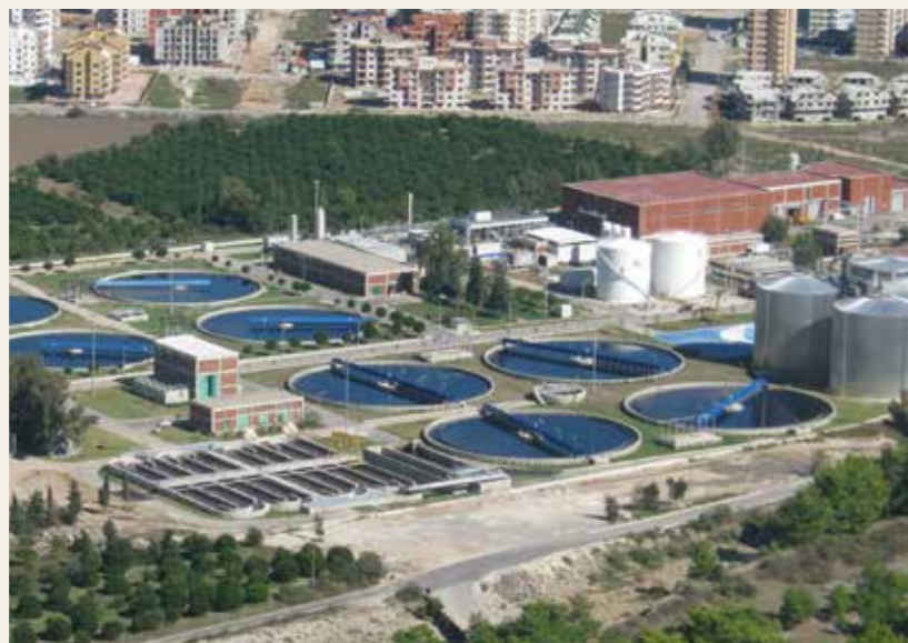
Antalya Hurma Wastewater Treatment Plant
