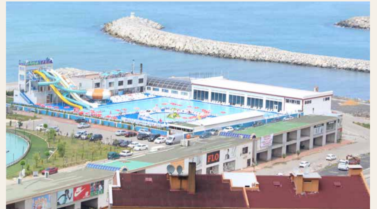
Zonguldak / Kozlu, Seaside Landscaping
