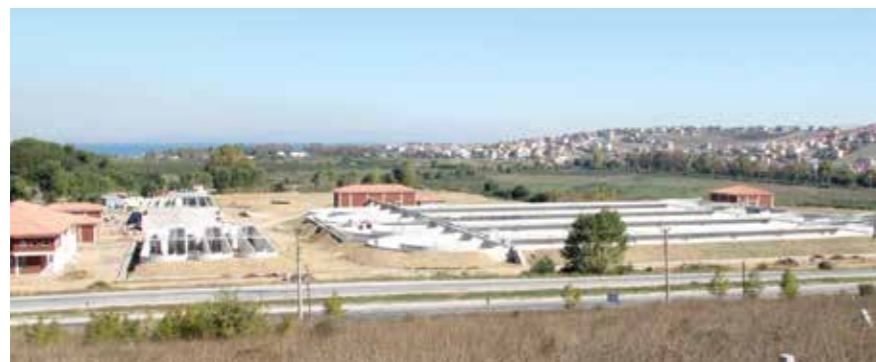
Yalova Advanced Biological Waste Water Treatment Plant
