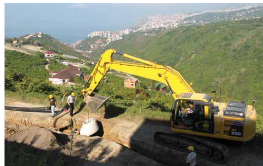
Trabzon, Akyazi Gürbulak Sewer System Construction Work
