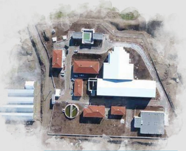
Adiyaman Kahta Drinking Water Treatment Facility
